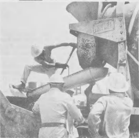
THREE READI-Mix trucks kept concrete hoppers, above, continually filled in the dawn to dusk operation. After a two-cubic-yard hopper, left, was filled, it was swung out to the dolphin by Raymond's big crane, lower left, and dumped in the steel reinforced base, lower right.
